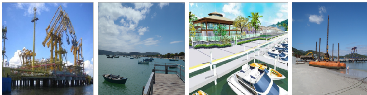
Figure 7. From right to left: (a) Assignment of public water bodies/Sea - Gasoduct in a marine platform; (b) assignment of public water bodies/Sea - Fishing pier in Bombinhas [SC]; (c) assignment of public water bodies/Sea - Marina in Balneario Camboriu [SC]; (d) assignment of public water bodies/Sea - ship Pier in Porto Belo [SC], Brazil.
