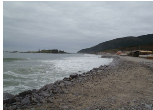
Figure 9. Building authorization-seawall made of stones in Florianopolis [SC], Brazil.
