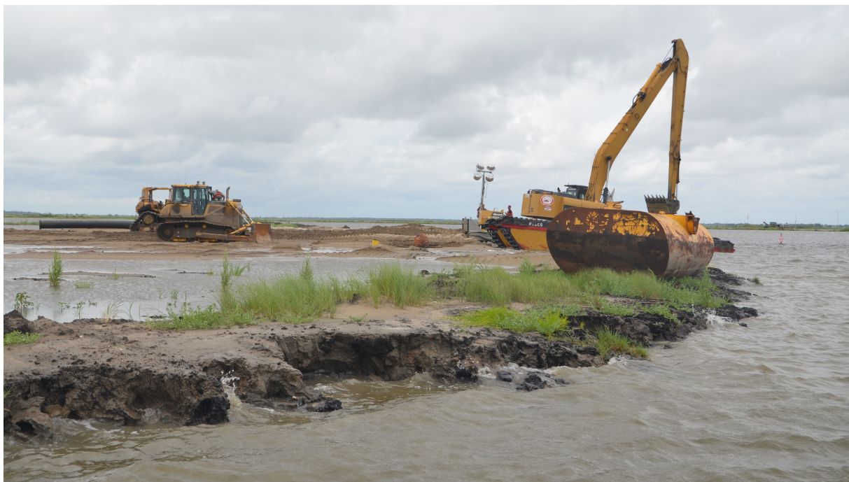
Figure 7. Land building using sediments dredged from the Mississippi River and piped as a slurry to the wetlands near Barataria Bay. This process is favored by local fishermen in contrast to the large-scale sediment diversions. Photo by author.
