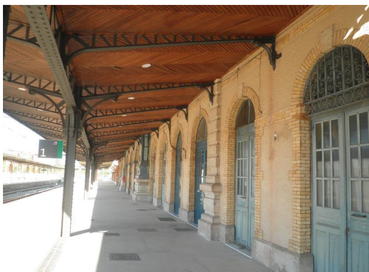
Figure 12. Rear facade canopy. Source: Morales Medina, 1987.
