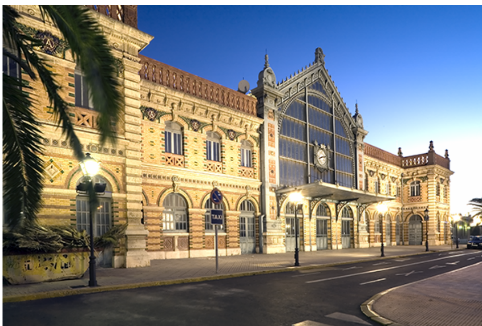
Figure 1. View of main facade of Almería Railway station.
