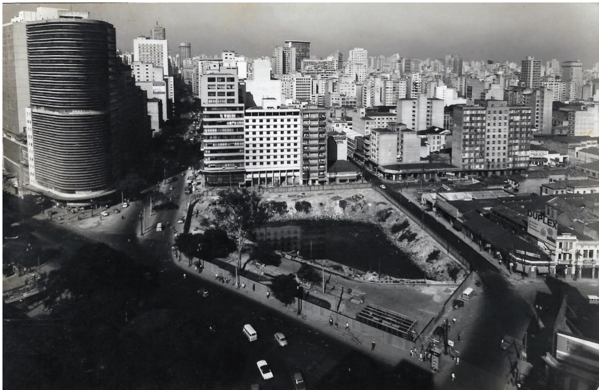
Figure 3. View of the plot where Alfredo Issa multistory parking garage was going to be built. Since the 1940s, with the abandonment of the works of the Security State Department, the place was abandoned and turned into an artificial lake, which caused lots of complaints. Collection: Benno Perelmutter Arq e Plan Ltda.
