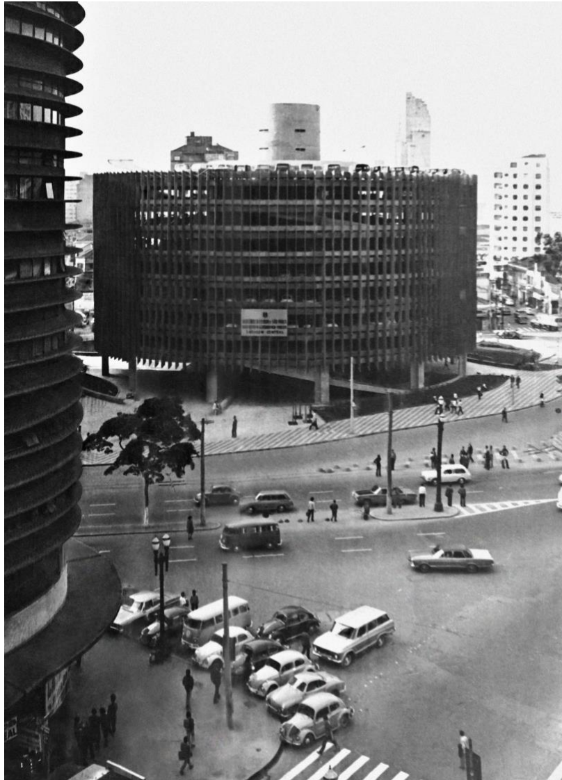
Figure 10. Alfredo Issa multistory parking garage recently built. Notice the visual integration of the entire surrounding area, the fluidity of public space and the square being actually used, with benches and other furniture. Collection: Benno Perelmutter Arq e Plan Ltda.
