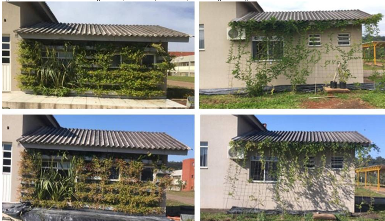
Figure 5 – Exterior view of vertical vegetation systems with plant development: living wall and green facade
