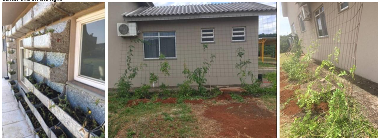
Figure 2 – Vertical vegetation systems on the planting day: living wall in the photo on the left (02/24/2022) and green facade (11/26/2021) in the center and on the right
