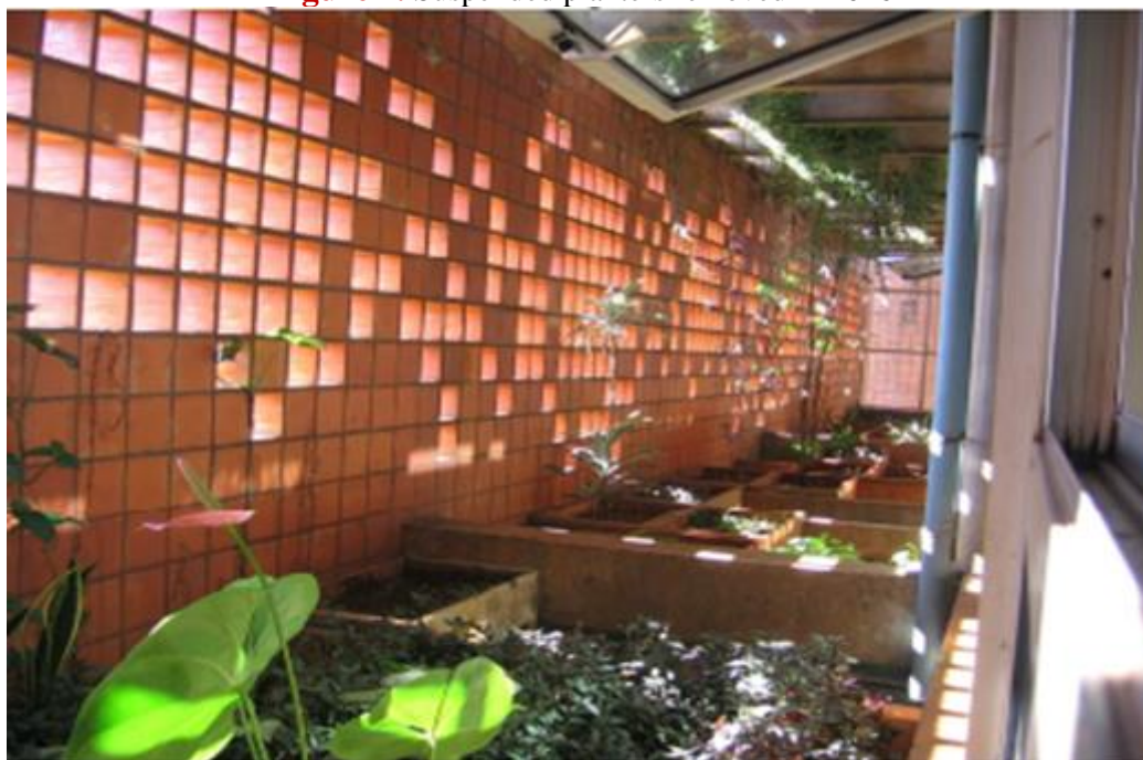
Figure 2. Suspended planters removed in 2016
